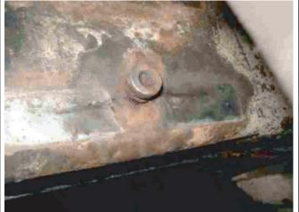
Over-torqued Clamping Hardware
